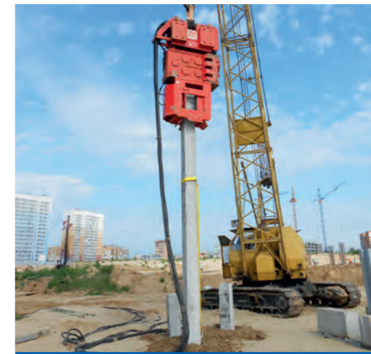
30HV Vibrodriver equipped with Multigrip clamp driving 350 mm square concrete piles in Russia.
